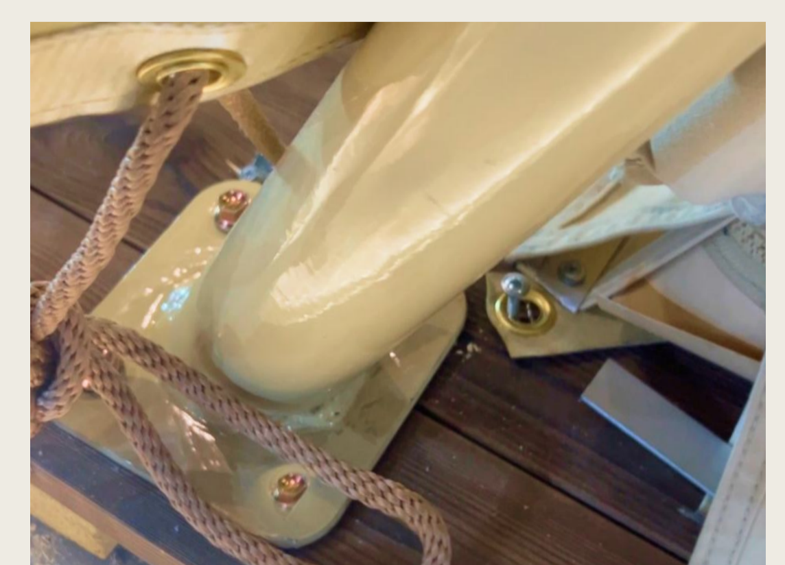
Ground Anchor Fixing
